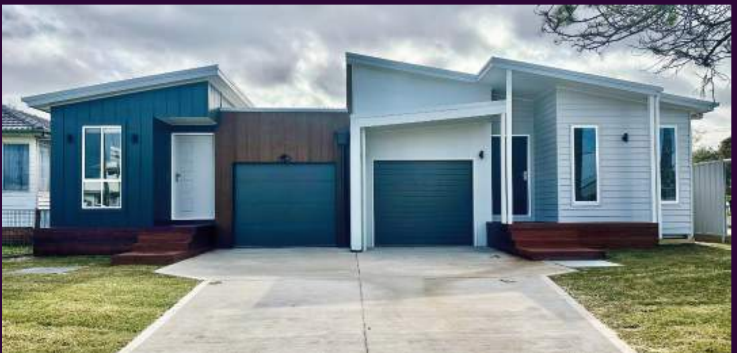
Belmont Project – Stage 1 Completion
